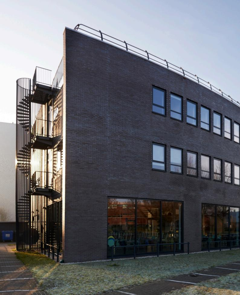
One of our Partners in The Netherlands was contracted for a large project, involving a combination of several XSGuardrail systems. The architect's main demand and concern was to keep the building's exterior completely intact. By installing specially coated guardrails, the systems are integrated into the building's design, minimizing the impact on its outer appearance.
